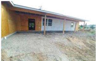
In the picture you can see the built-up grade at the front porch, as well as the posts that require elevated.
