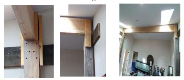
In these pictures it can be seen that the glulam beam and 8x8 posts have been adjusting to the continuous changes in the post & beam foundation support. It appears from the outside that the front room is trying to pull away from the rest of the house. This is the wall that had the window break due to compression a few months ago. The whole support system can be seen below.
