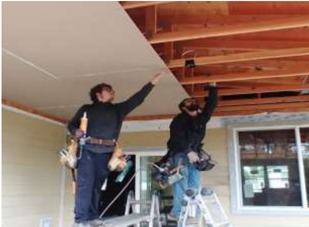
Seth (left) & Ford (right) installing back porch ceiling panels
