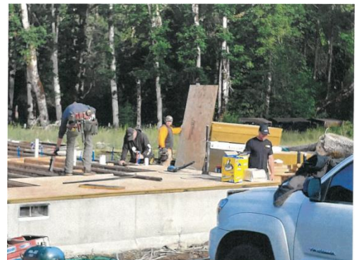
Coast Fork Construction laying down sub-flooring
