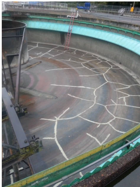
Repairs to the concrete skin coat on the bottom of clarifier number one.
