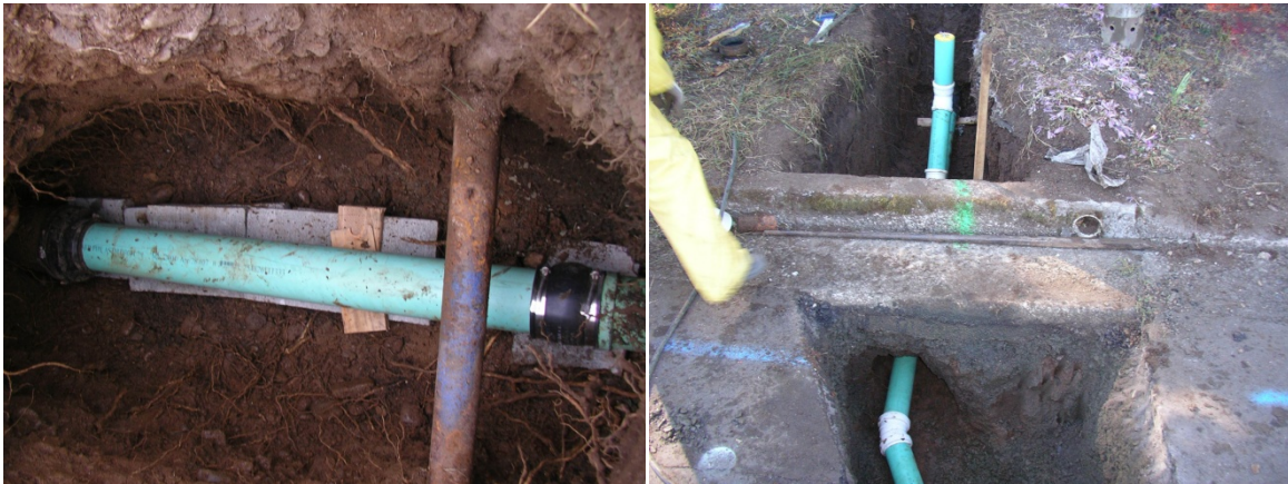
Left – August 20, 2012 – Sanitary lateral repair at 1148 South 4 th Street.
