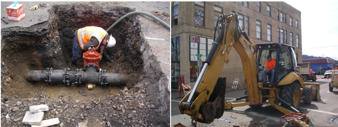
Installation of new 8" gate valve at 8th and Main – April 8, 2013
