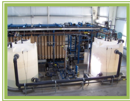
A portion of the Micro-Filtration Membrane at the Row River Water Treatment Plant
