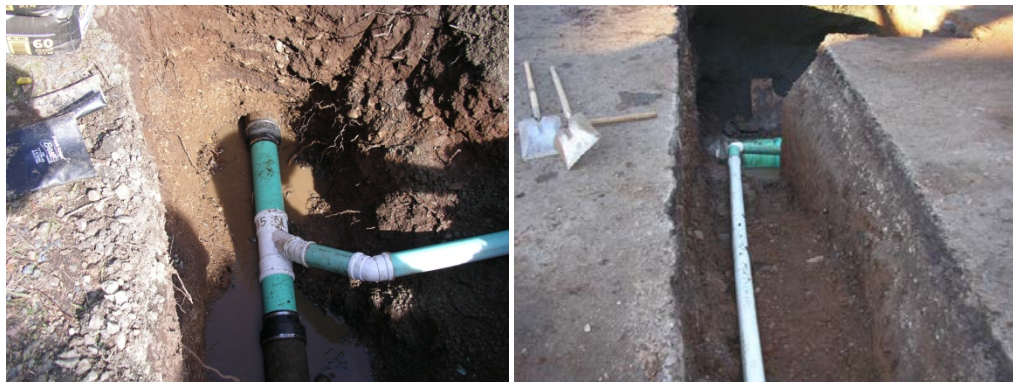
Left – March 8, 2012 – Replacement of failing sanitary lateral line 647 1 st Street.
