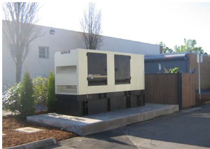
Emergency backup 150 kW Kohler Generator at City Hall
