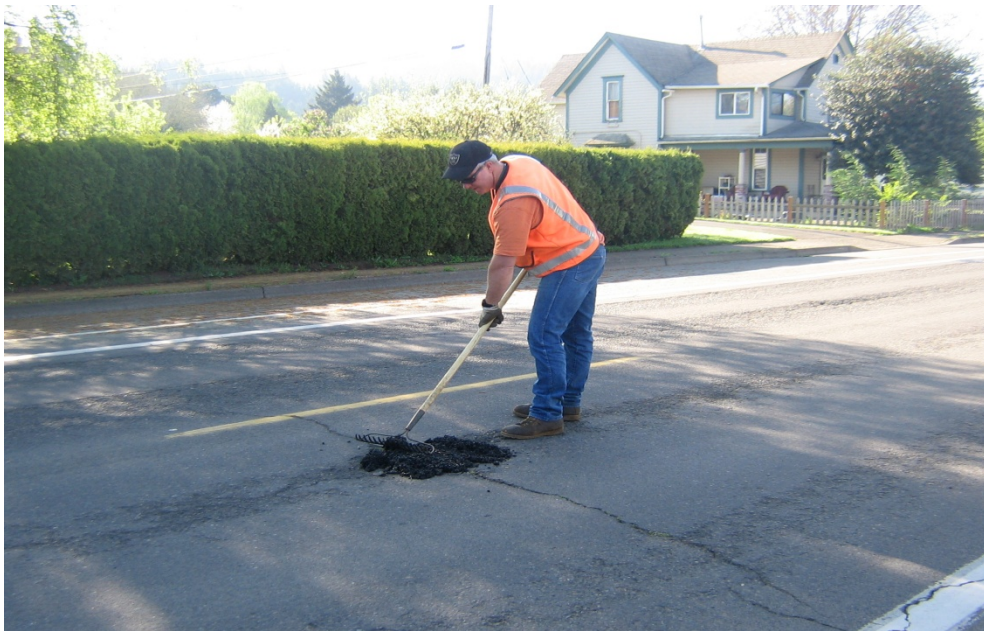
Patch repair on South 6 th Street, April 23, 2012.
