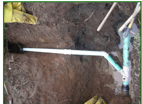
March 1, 2011 – Replacement of failing sanitary sewer lateral line at 1031 Washington Avenue.
