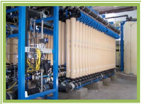
A portion of the Micro-Filtration Membrane at the Row River Water Treatment Plant
