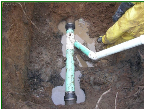
March 1, 2011 – Replacement of failing sanitary sewer lateral line at 1031 Washington Avenue.
