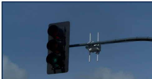
A Cisco wireless radio which transmits the WiFi signal, is mounted to a traffic light.
