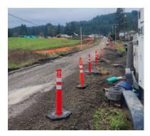
Delta Construction finished the temporary access road to 4<sup>th</sup> Street and is making progress in placing the 10" water line from 6<sup>th</sup> Street to the west on Cleveland Street.
