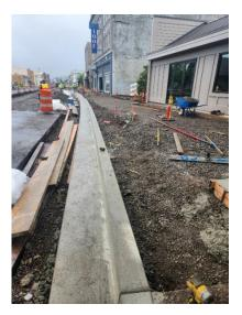
The excavation along 5th Street, from Main Street to Rainy Peak Bike Shop is finished. The team is currently leveling the area to prepare for the installation of curb forms needed to pour the curb, gutters, and a 4-foot section of the sidewalk.
