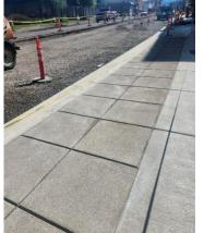
The area on 7th Street, next to All America Square, is planned to become a festival street. The storm drains, electrical, and irrigation conduits have been installed. Preparations have begun to frame the curb and gutter.
