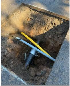
This morning, at 8:00 AM, Public Works was alerted to a water leak in the 700 block of S. 16th Street. Upon investigation, it was determined to be a 6-foot cast iron water mainline break.
