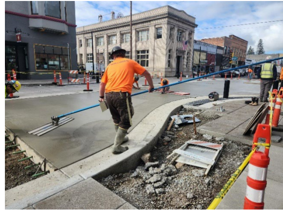
Intersection at 6 th and Main
