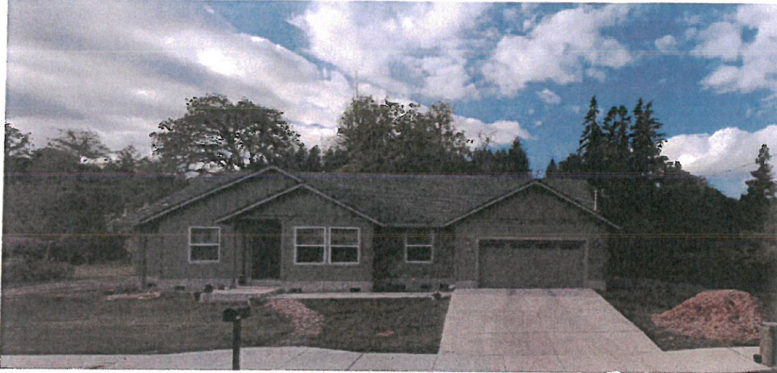
New construction (2014). Note all the flood openings!
