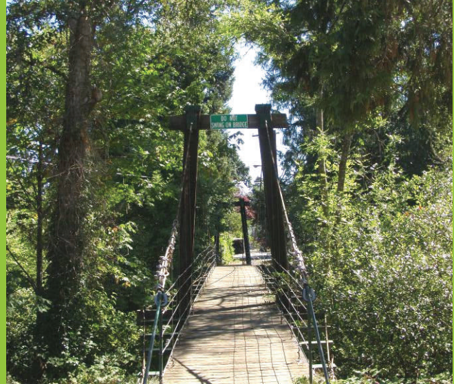
Swinging Bridge over Coast Fork of the Willamette River.
