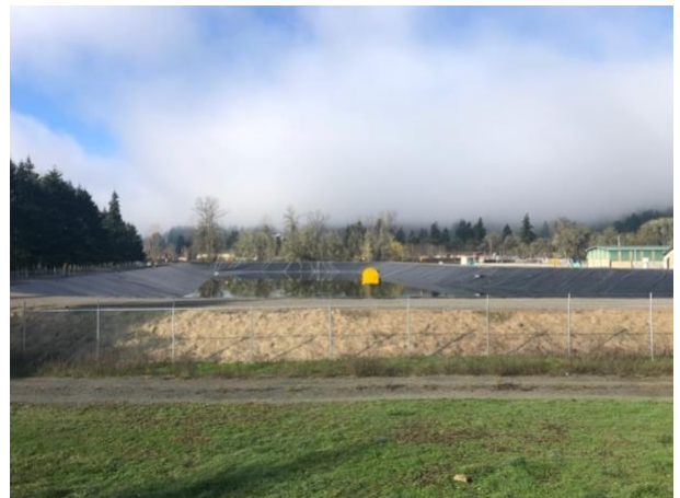
Completed Effluent Water Pond, December 2020
