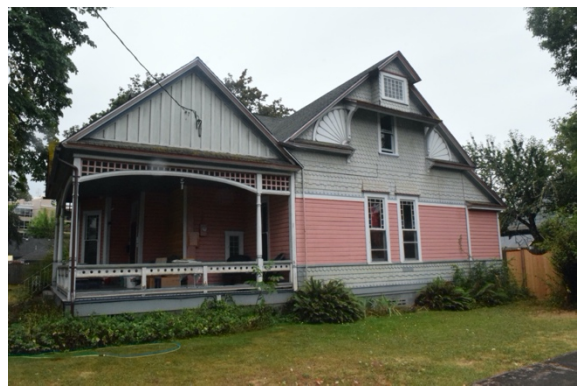
4. View to south from Ash Avenue. 2020.
