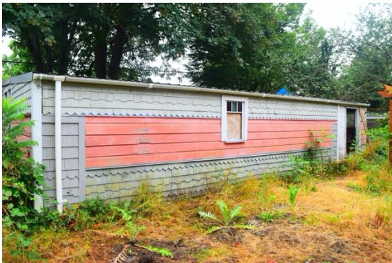
5. Storage shed outbuilding. 2020.
