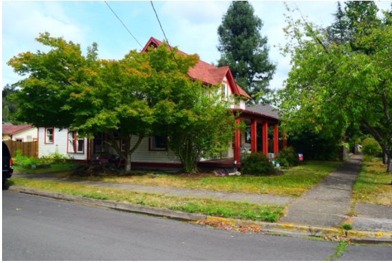
1. View to northeast from intersection of North L St. and Ash Avenue. 2020.
