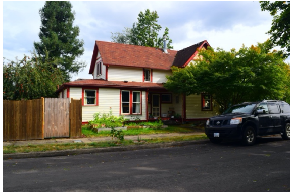
2. View to east from North L Street. 2020.
