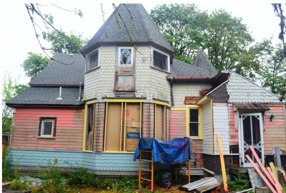
3. View to east from rear of property. 2020.
