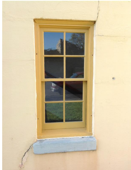
Restored window at the Cottage Grove Armory.
