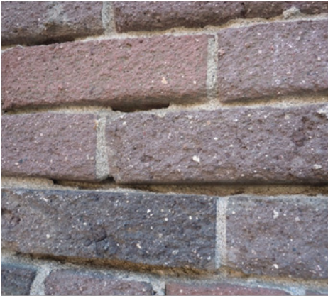
Fig. 26 Effects of abrasive cleaning on brick and mortar
