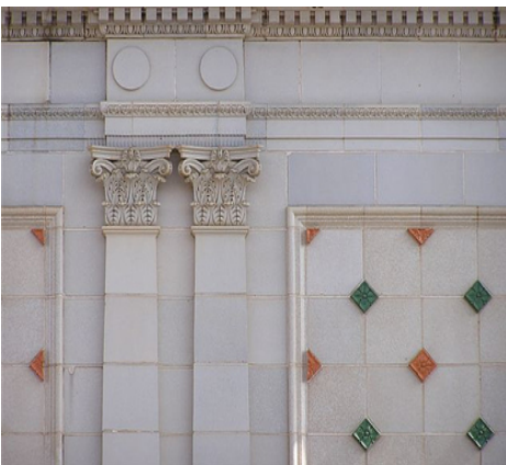
Figure 4. Ceramic Veneer and Glazed Architectural Terra Cotta. ( http://concretecircles.blogspot.com )
