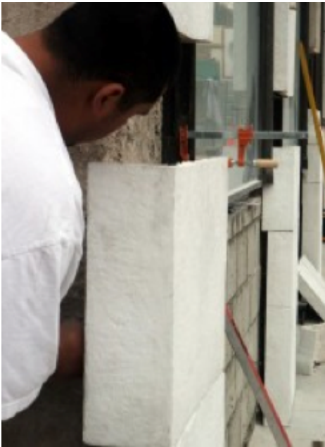
Figure 19. Anchoring of a replacement Terra Cotta Unit (www.preservationarts.net)
