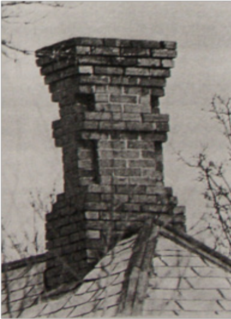
Fig. 3 Chimney by Wallace, Cottage Grove, 1890 (Dole 1983, 21)
