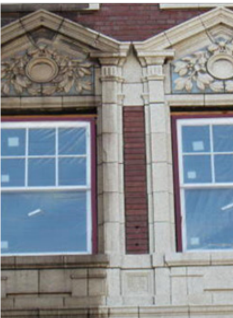
Figure 16. Cleaning Architectural Terra Cotta (www.preservationarts.net)
