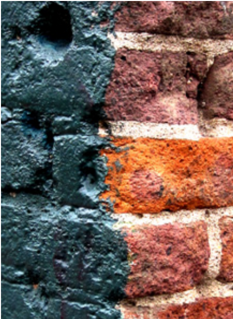
Fig. 10 Historic masonry that has been continually painted and maintained
