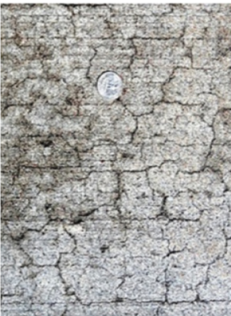
Map Cracking
