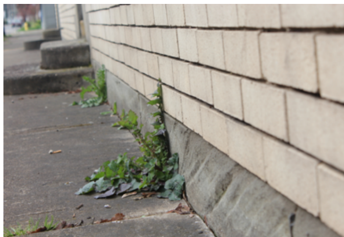
Figure 7: First National Bank Building – Stone
