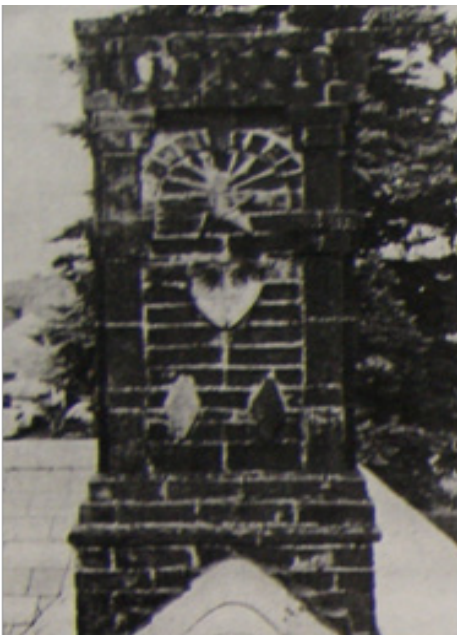
Fig. 4 Chimney by Wallace, Springfield, 1873. (Dole 1983, 20)
