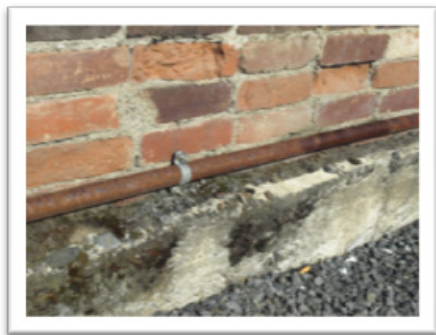
Poor Consolidation: Aggregate Ratios
