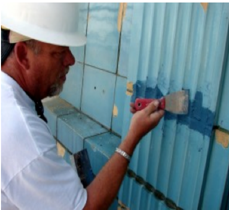
Figure 22. Repointing procedure ( www.preservationarts.net )
