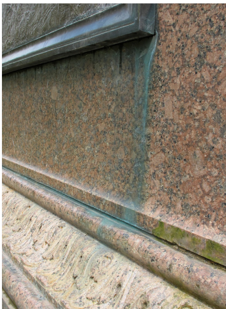
Figure 15: Copper staining, biological growth and missing mortar on the Pioneer Mother Statue require some attention before they become truly problematic for the stone
