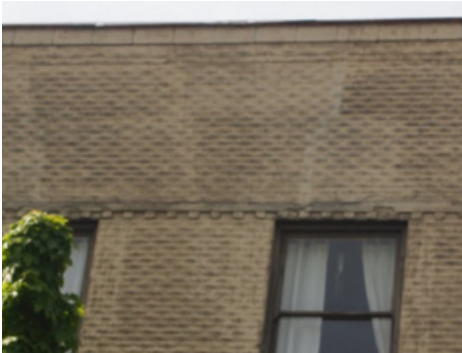
Figure 6: Water Damage
