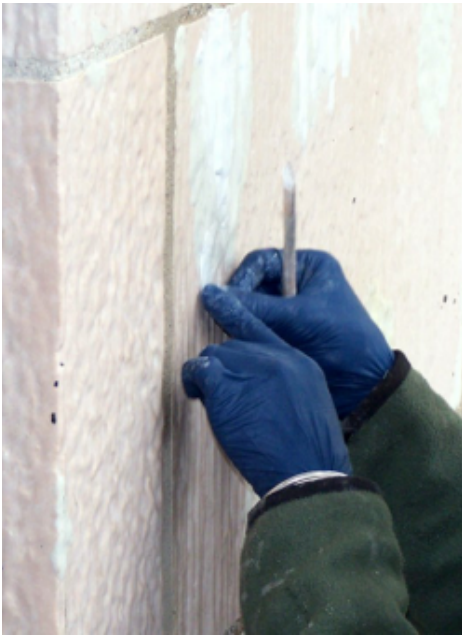
Figure 17. Coating Repair on a Glazed Terra Cotta Unit (www.preservationarts.net)
