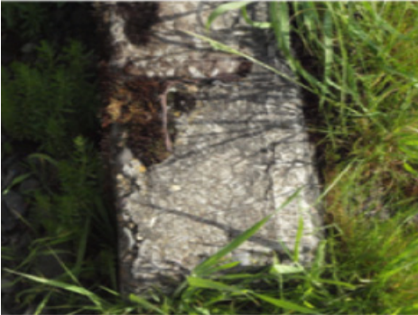
Cracking: Corrosion
