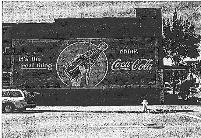
Brick that was not historically painted should remain bare, however, any historically painted brick, like the above Coca-Cola sign, should be preserved.
