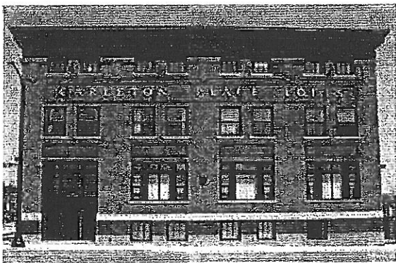
Carlson Place (historic name: Simmons Manufacturing Company), St. Paul, Minnesota (1909). Before and after rehabilitation for residential use. Courtesy Hess, Roze and Company
