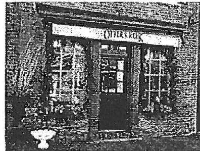
Appropriate lettering, as on this roller awning valance, can function as distinctive signage without detracting from the historic character of the building. Photo: NPS files.
