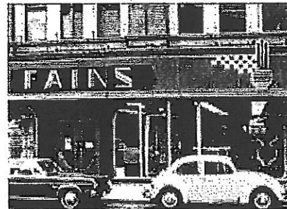
This 1930s Moderne storefront has gained significance over time and should be preserved. Photo: NPS files.
