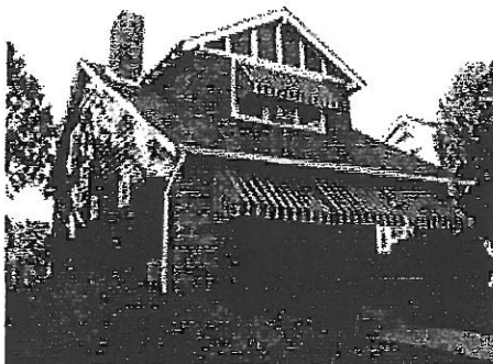
Simple shed-type awnings with acrylic or canvas coverings and free-hanging valances are appropriate for most historic residences featuring rectilinear openings. Photo: NPS files.
