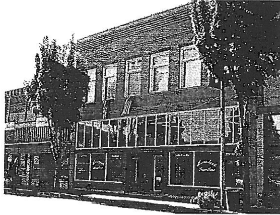
The newly redone Homestead buildings display rhythm with their first and second floor windows.
