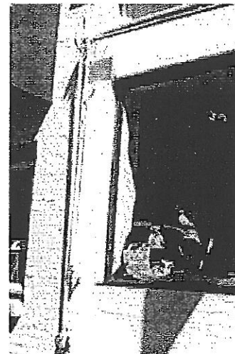
A gearbox, slide rod, roller, front bar, and extension arm reveal that this 19th century facade once featured a retractable awning. It is likely that with minor repairs the
