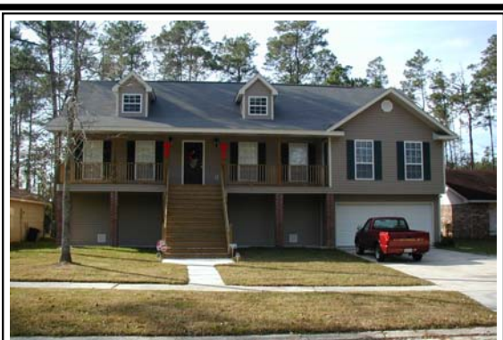
This house in St. Tammany Parish was elevated with funding support from DHS/FEMA. The owner paid the 25% non-Federal share. The Parish amended its zoning ordinance to measure the height restriction from the 100-year flood elevation, rather than from the ground, facilitating elevation projects for taller buildings.
