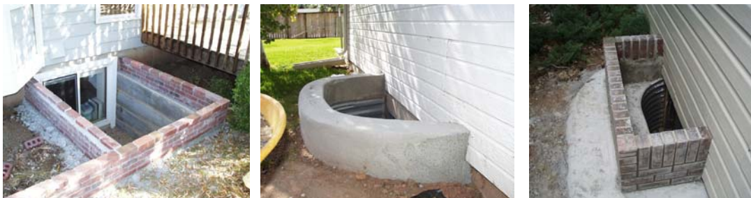
Some of Fort Collins' flood proofing projects to keep surface waters from entering basements
