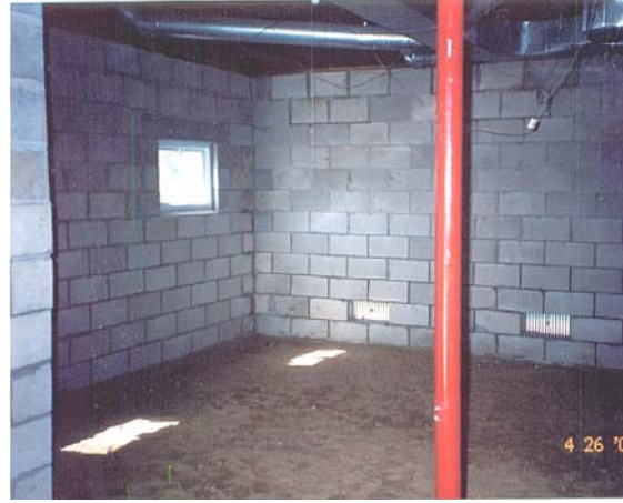
These houses in Vassar, Michigan, illustrate two approaches to elevating. The one on the left had the foundation backfilled and landscaped to minimize the adverse appearance of an elevated building. The one on the right left the lower area open, but included vents to allow water in to equalize hydrostatic pressures. The interior is bare and built of water resistant materials. However, over the years, the owner may be tempted to finish this area with carpeting, wallboard, and other materials subject to flood damage.
