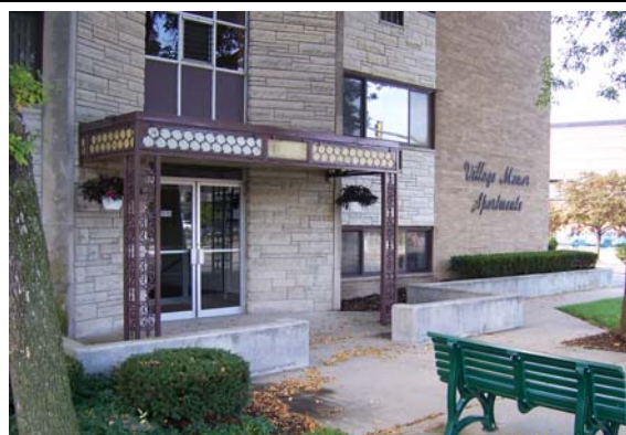
The floodwall on the left was built by Rosemont, Illinois, to protect a Village owned housing project. Note that sandbagging is required to close the opening at the sidewalk. The site has 24-hour maintenance crews, stockpiles of filled sandbags, and a warning system, so human intervention has not been a problem. The floodwall on the right is in Fort Collins, Colorado. It has a steel doorway that stays closed, so it does not depend on human intervention.
