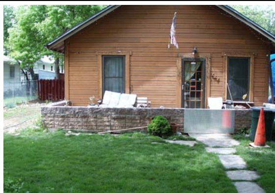
The floodwall on the left was built by Rosemont, Illinois, to protect a Village owned housing project. Note that sandbagging is required to close the opening at the sidewalk. The site has 24-hour maintenance crews, stockpiles of filled sandbags, and a warning system, so human intervention has not been a problem. The floodwall on the right is in Fort Collins, Colorado. It has a steel doorway that stays closed, so it does not depend on human intervention.
