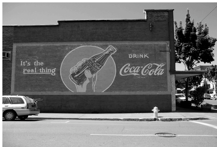
Brick that was not historically painted should remain bare, however, any historically painted brick, like the above Coca-Cola sign, should be preserved.
