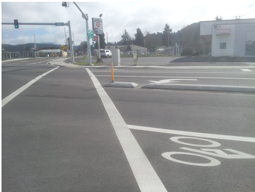
Roadway Striping on OR 99
