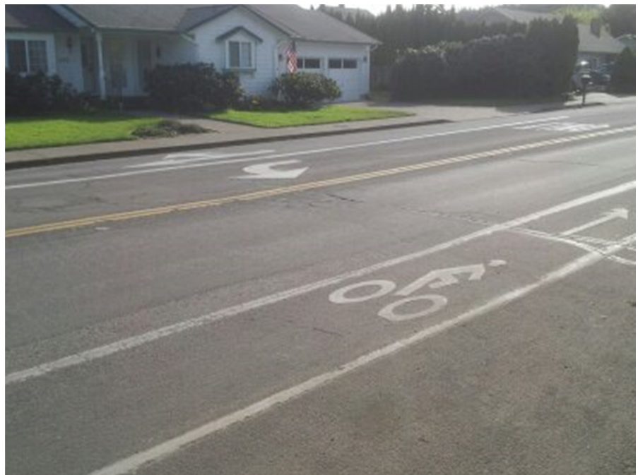
Bike Lane Striping
