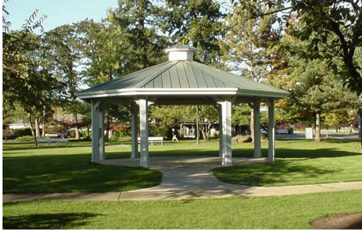
Coiner Park Gazebo, rebuilt in 2003
