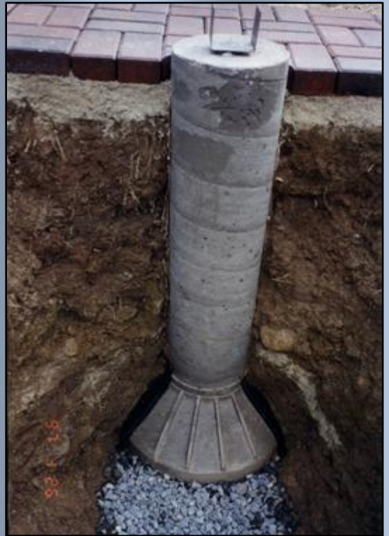
A concrete pier footing. This demonstrates the construction of this BMP.
