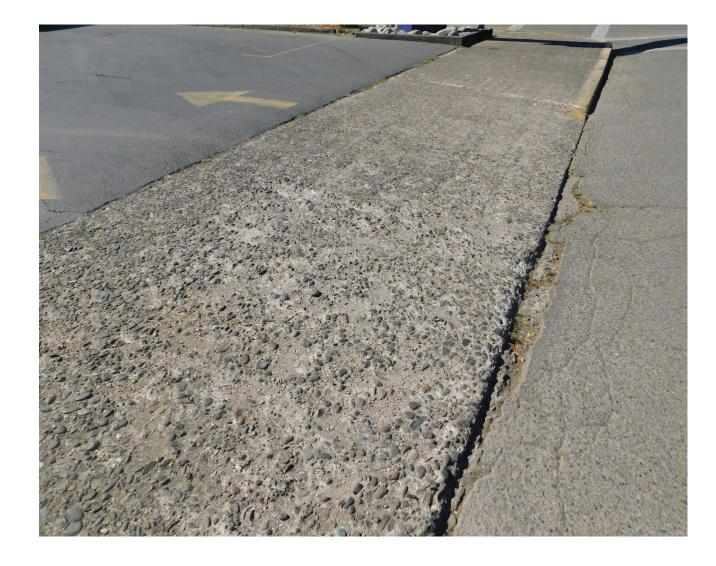
Example of Extremely Uneven Concrete & Tree Upheaving Sidewalk
