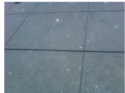
Select concrete paving along Main St. could include a silica sand mixture, which gives the pavement a subtle sparkle, especially visible at night.
