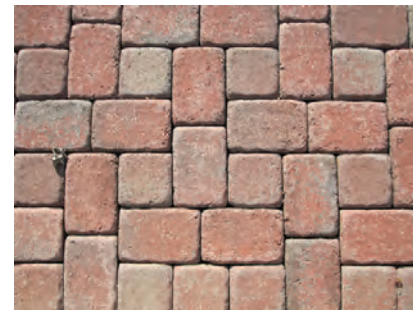
Concrete unit pavers in a simple offset pattern and a warm reddish brown color are proposed for crosswalks and the festival street on 7th. Fields of pavers would be bordered by concrete for ease of maintenance.
