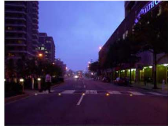
Embedded Pavement Lighting
