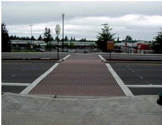
Textured Crosswalk with Pavers
