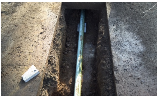
Left – Sewer line replacement, 636 South 2 nd , March, 2016.
