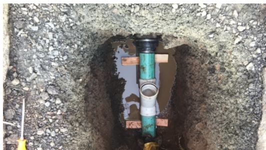
Left – Sewer line replacement, 636 South 2 nd , March, 2016.
