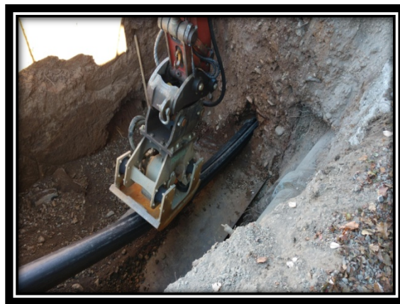
Pipe bursting new 6" sewer line to replace old 6" concrete line
