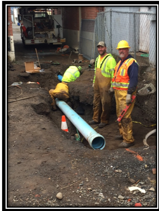
Installing a new storm line and catch basins
