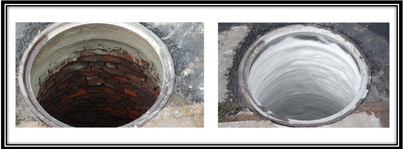
Old brick lined manhole on sealed to keep storm water from entering sewer collection system
