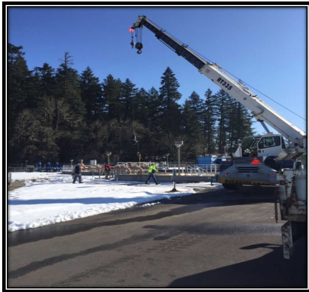
Craning in rebuilt motor for clarifier
