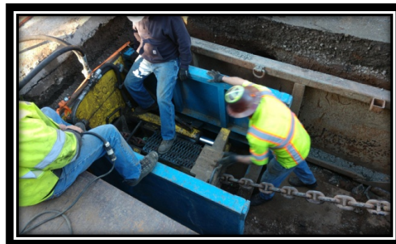
Contractor pulling in new 6" sewer line
