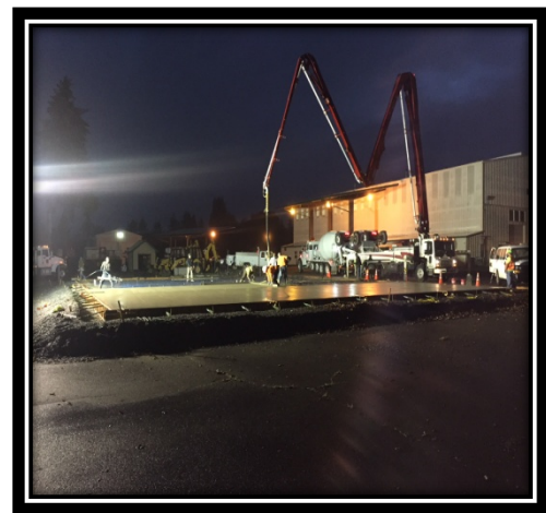
Pouring Concrete for new shop building
