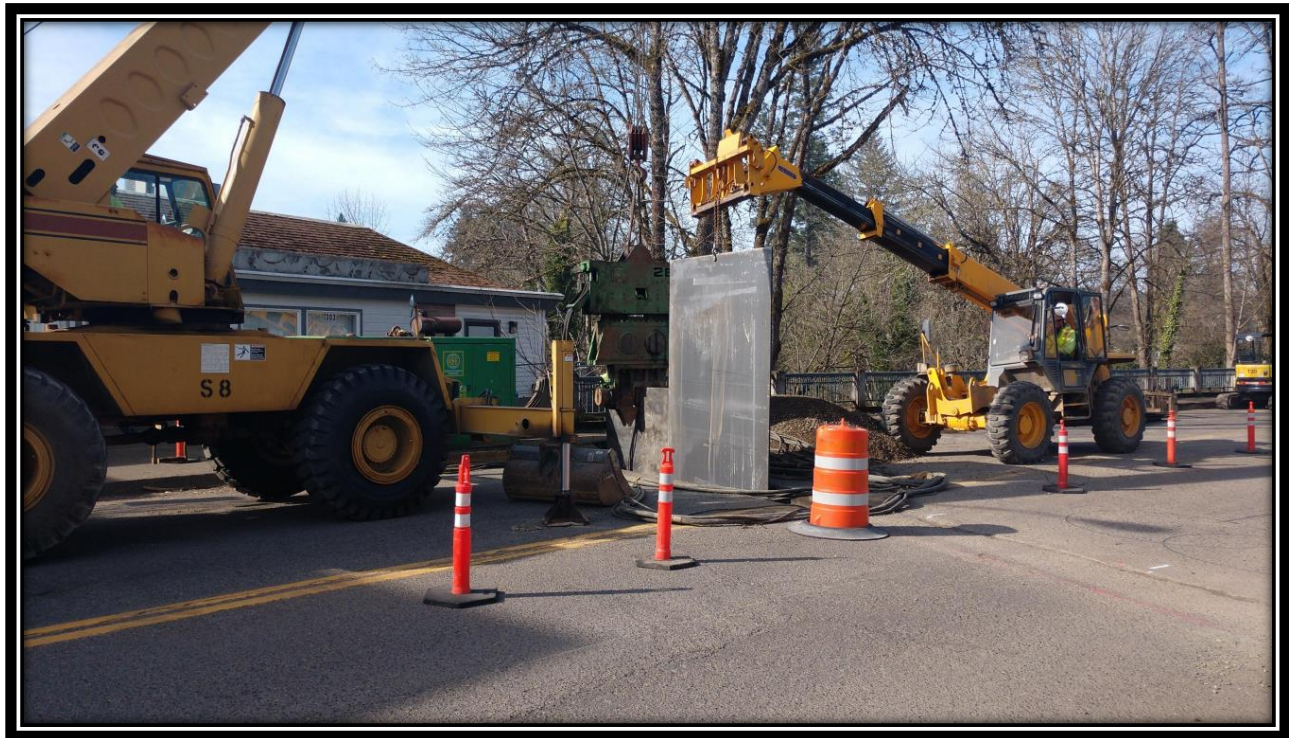
Installing new steel plates at the Main Street Bridge across the Coast Fork River
