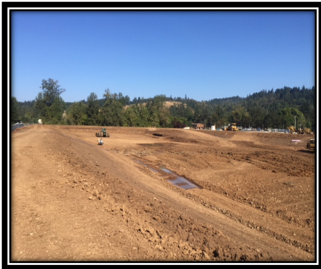
Construction of new effluent pond
