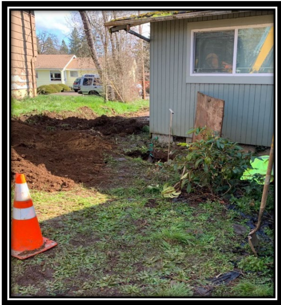
Sink hole caused by sewer mainline failure
