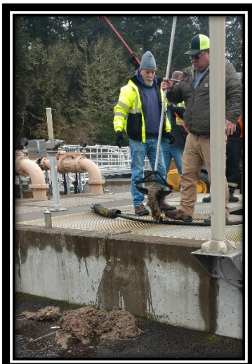
Sewer Treatment Plant plug from disinfecting wipes and rags
