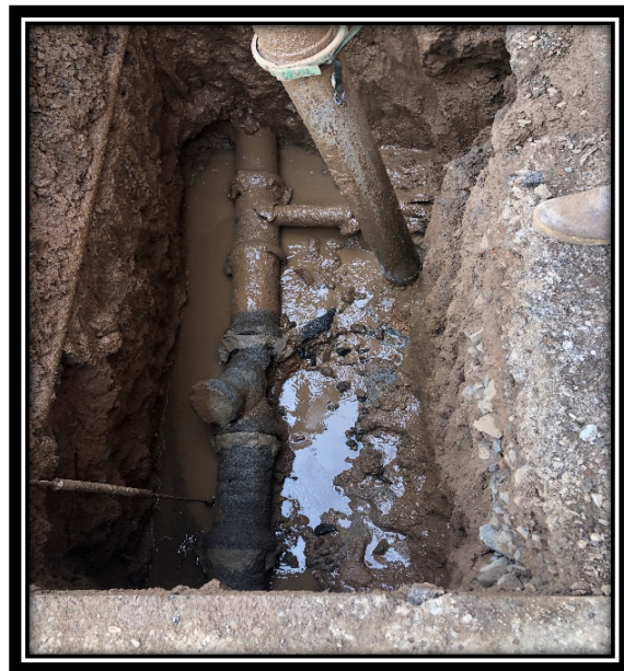
Sewer mainline repair
