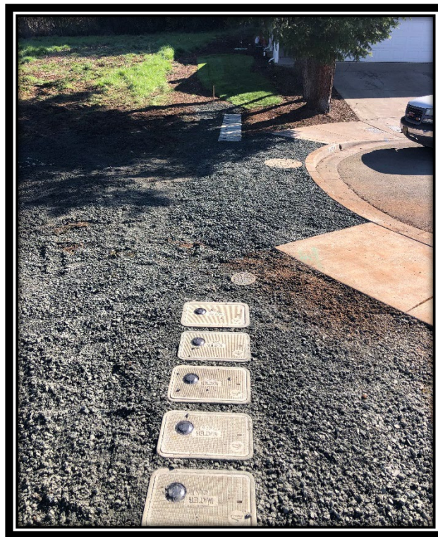
New water meter installation for 14 new townhomes
