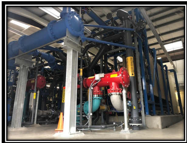
New 2 MGD Pall Filtration Rack
