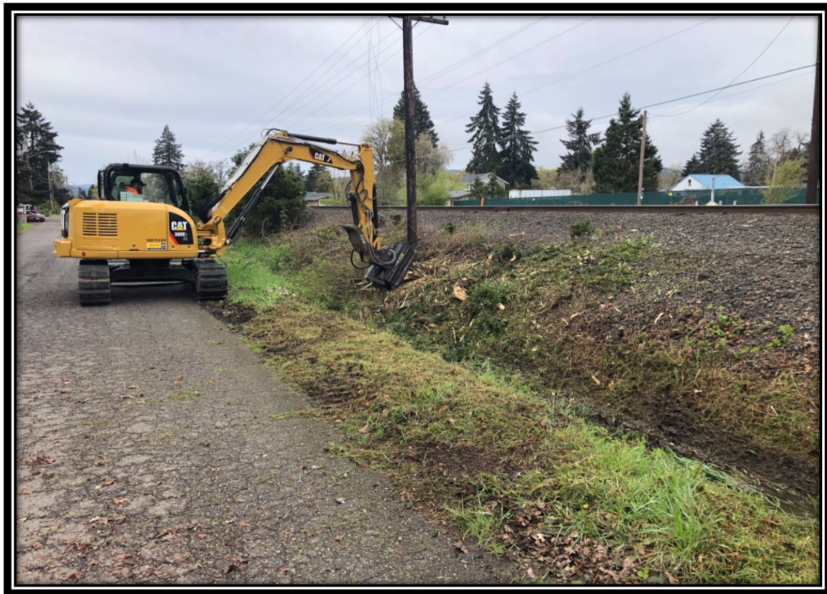
Brush cutting the storm drainage ditch along Douglas Street
