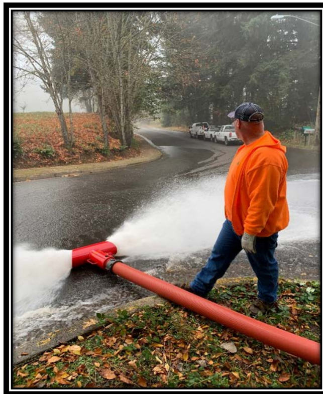
Flushing the water distribution system
