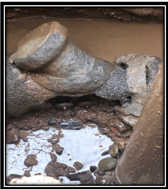
Wore out sewer mainline where video camera was stuck
