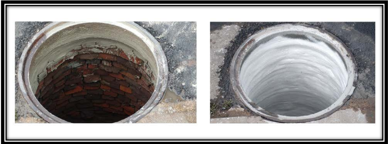
Old brick lined manhole sealed to keep storm water from entering the sewer collection system. In 2019-2020 the City contracted to have 15 sewer manholes to be repaired and sealed.
