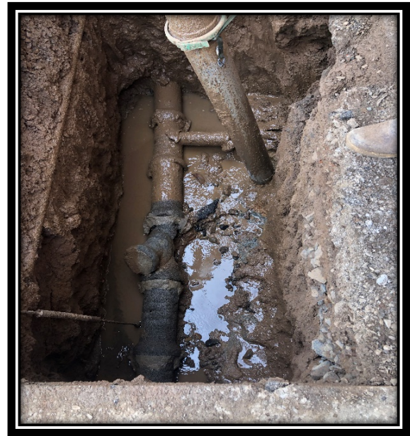
Sewer mainline repair
