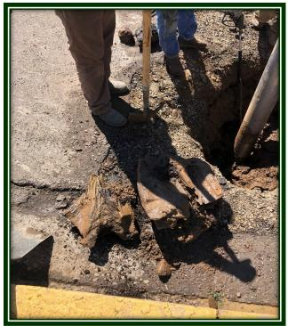
Sink hole on Gibbs caused by a rotten stump
