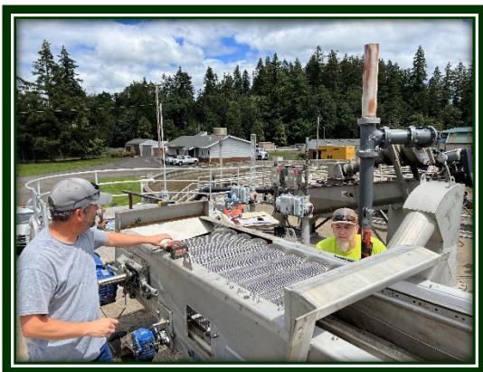
Staff rebuilding head works bar screen
