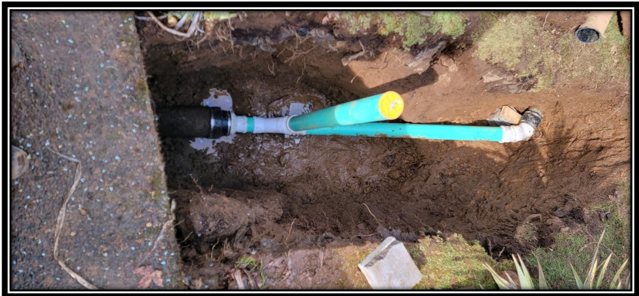
Lateral sewer line repair
