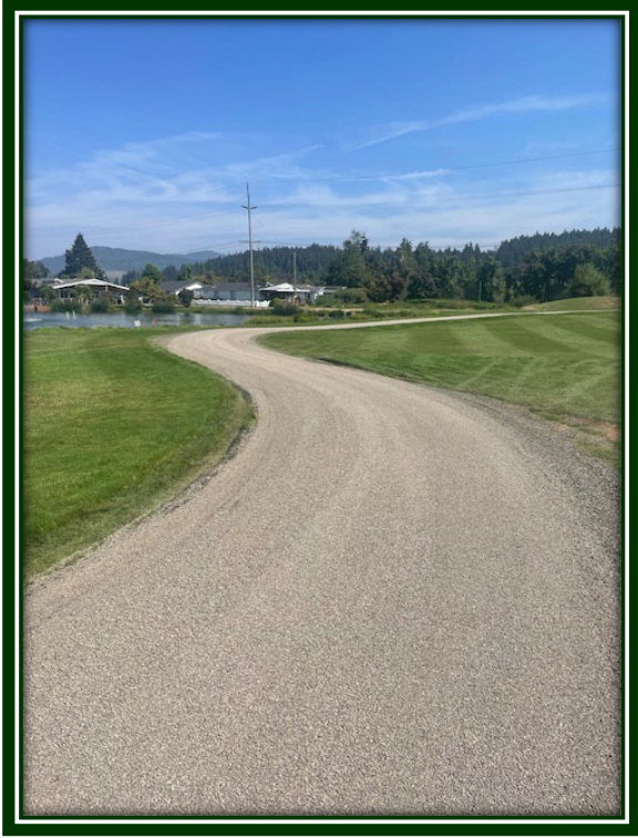
Chip Seal Hole #10 Cart Path
