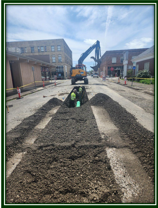
Main Street Revitalization Project New Storm Drain Line
