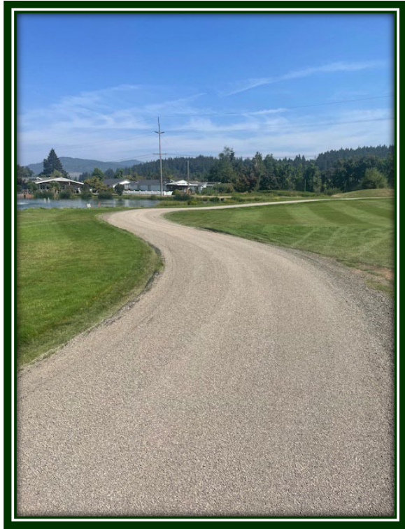
Chip Seal Hole #10 Cart Path
