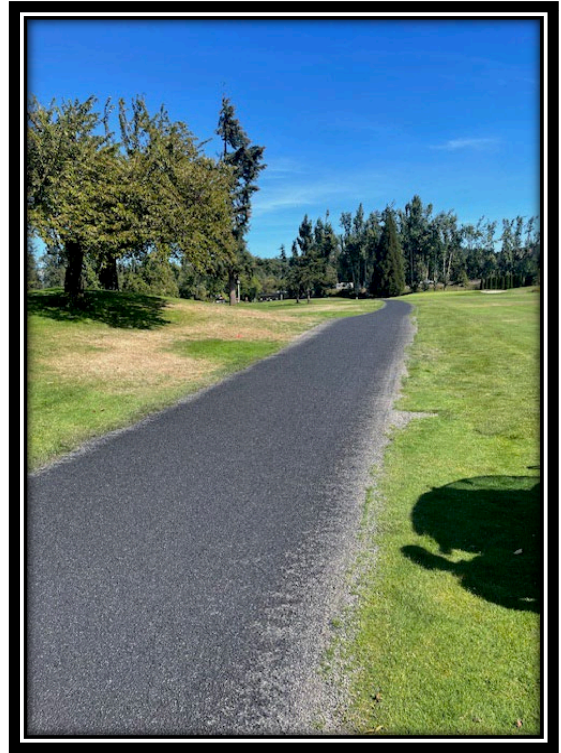
Chip Seal & Seal Coat on Hole #4 Cart Path
