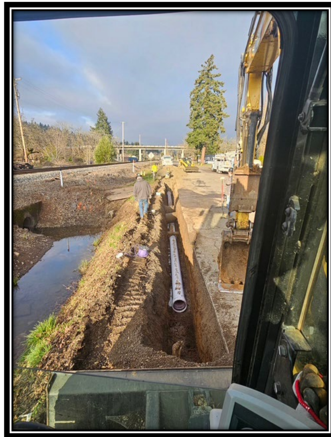
Installation of new 12" effluent line in Douglas Street
