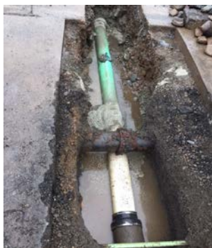
Sewer Line repair at Oswald West
