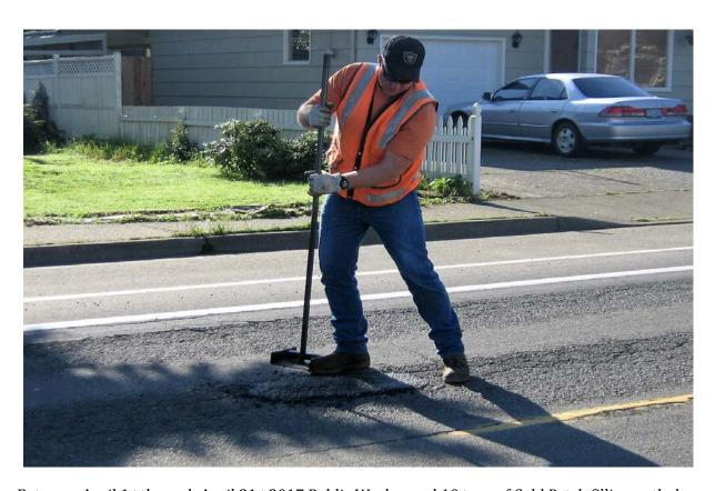
Between April 1st through April 21st 2017 Public Works used 10 tons of Cold Patch filling potholes.
