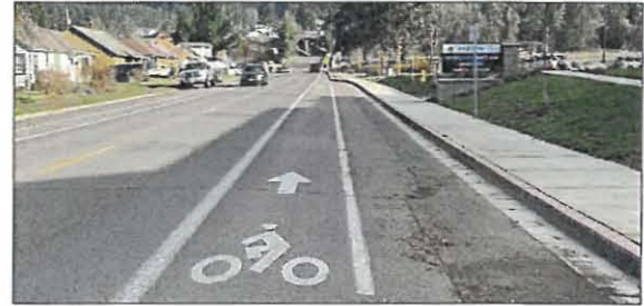
Figure 2-11. Typical Conventional Bike Lane
