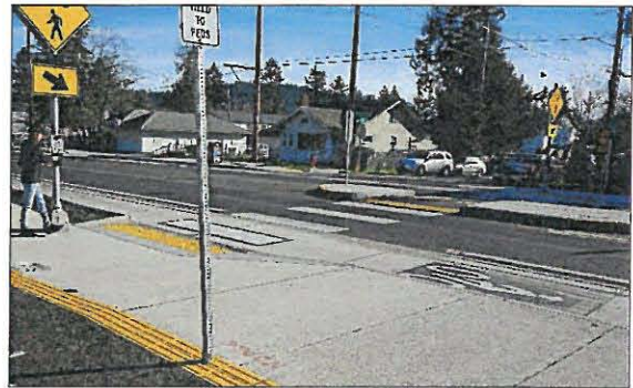
Figure 2-5. Typical Enhanced Crossing with Median
