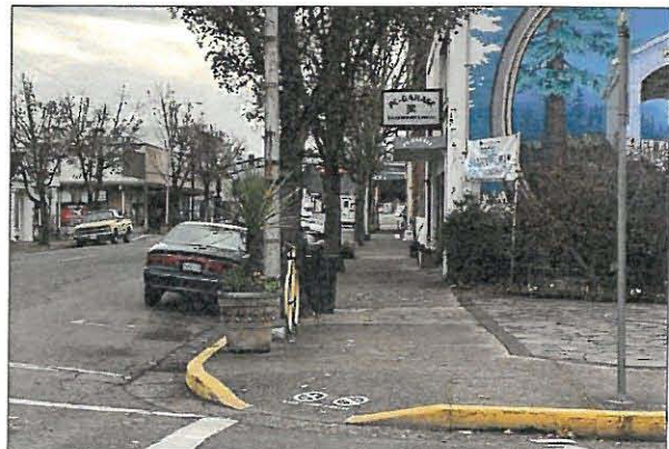
Figure 3-1. Sidewalk on W Main Street in Downtown Cottage Grove
