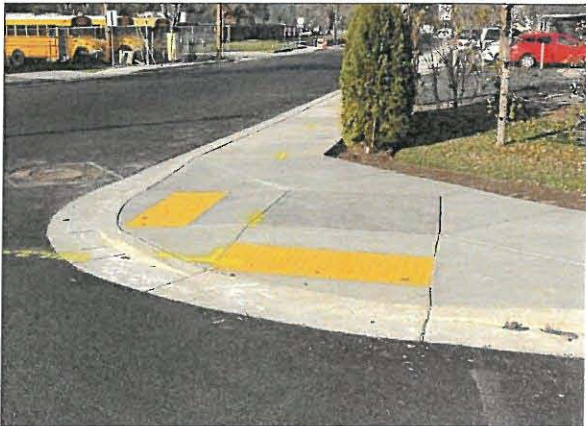
Figure 3-9. Recently Upgrade Curb Ramps near Lincoln Middle School
