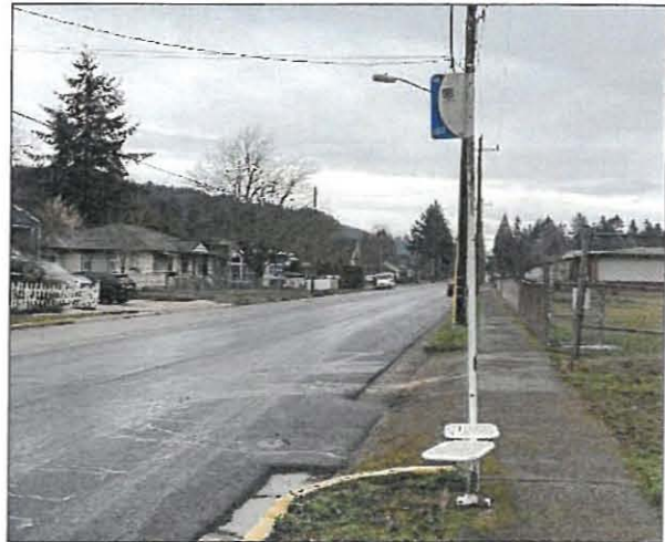
Figure 4-2. Typical LTD Route 98 Bus Stop
