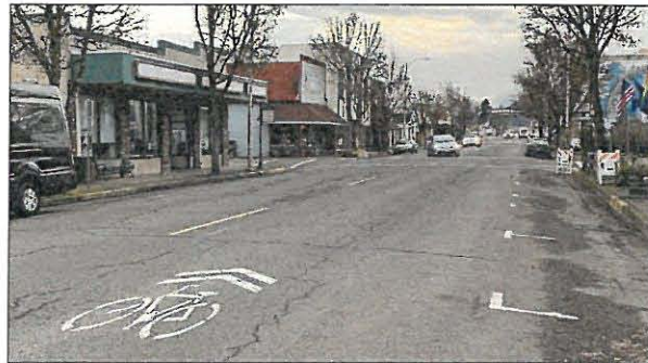
Figure 3-14. Typical Shared Roadway
