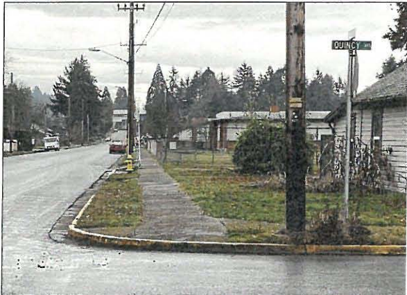
Figure 3-8. Missing Curb Ramps along Quincy Avenue
