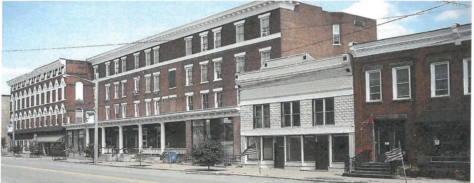
Essex County, NY - Town of Moriah, Hamlet of Port Henry. Main Street, Van Ornam & Murdock Block. Credit: Alex Scrodin
