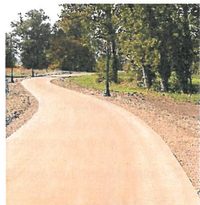
New Concrete Path and Light Poles on the South Bank Path
