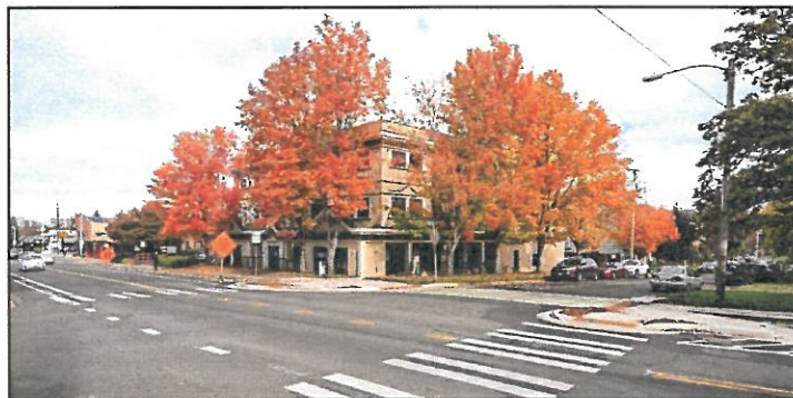
Completed Paving on 19 th Avenue
