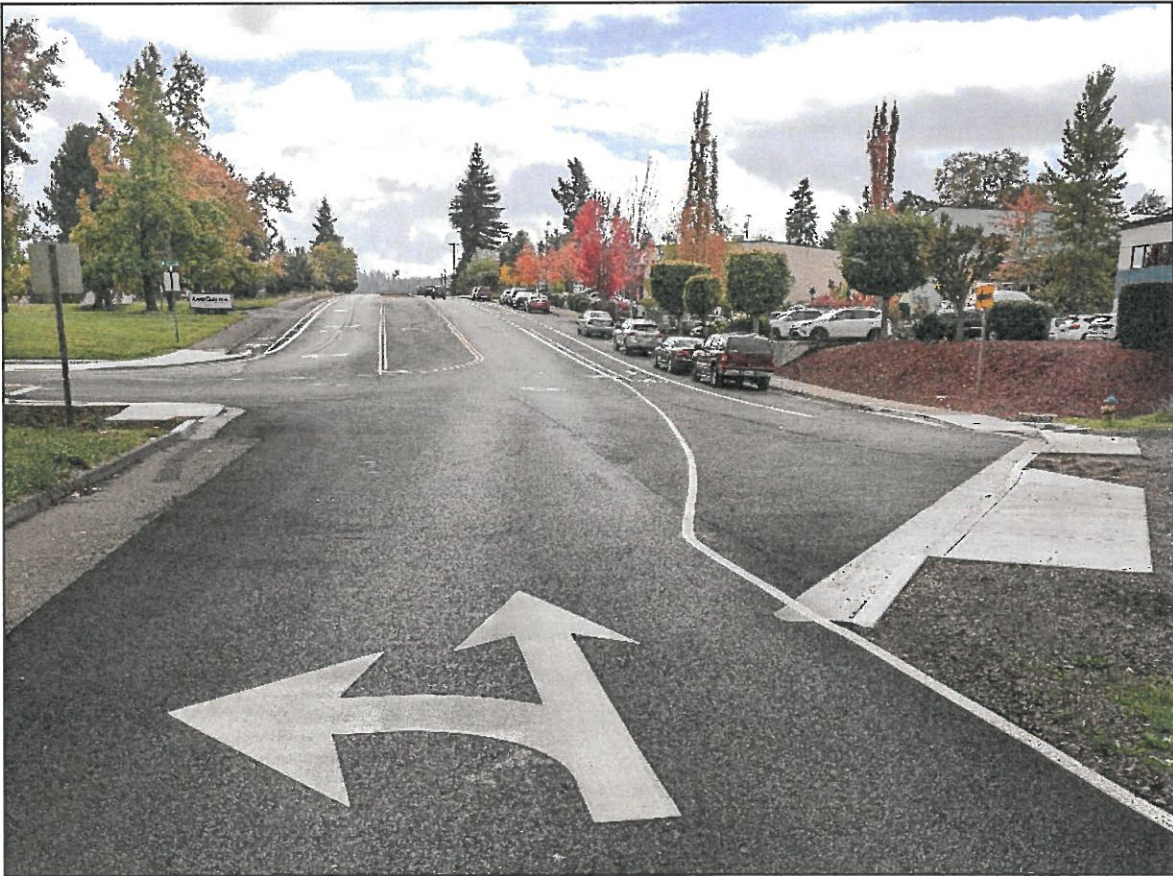
Completed Paving on Bailey Hill Road
