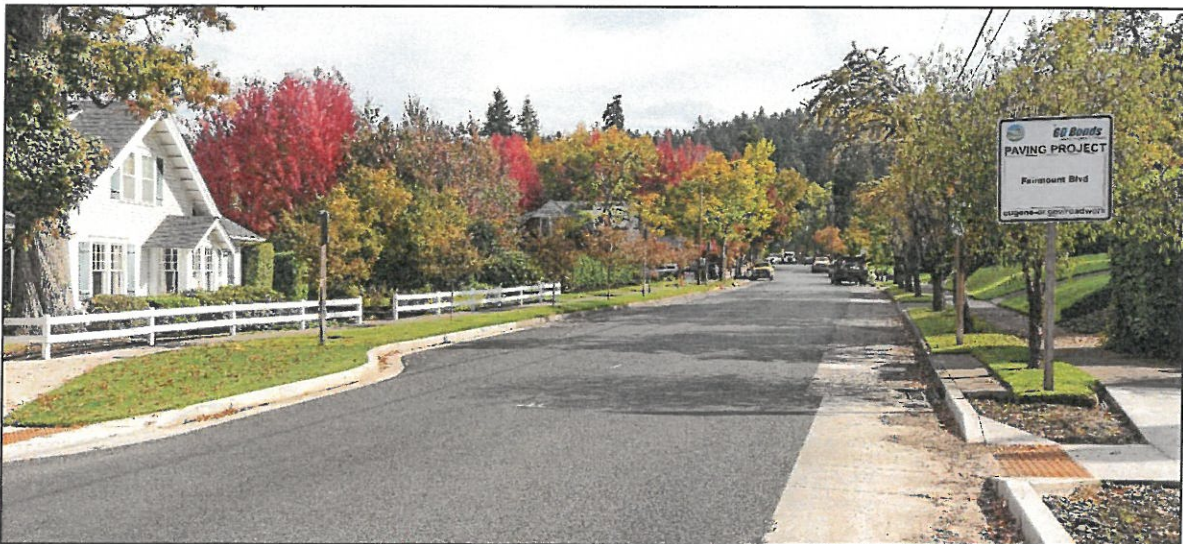
Completed Paving on Fairmount Boulevard
