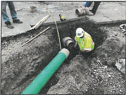
Stormwater Pipe Work on Primrose Street
