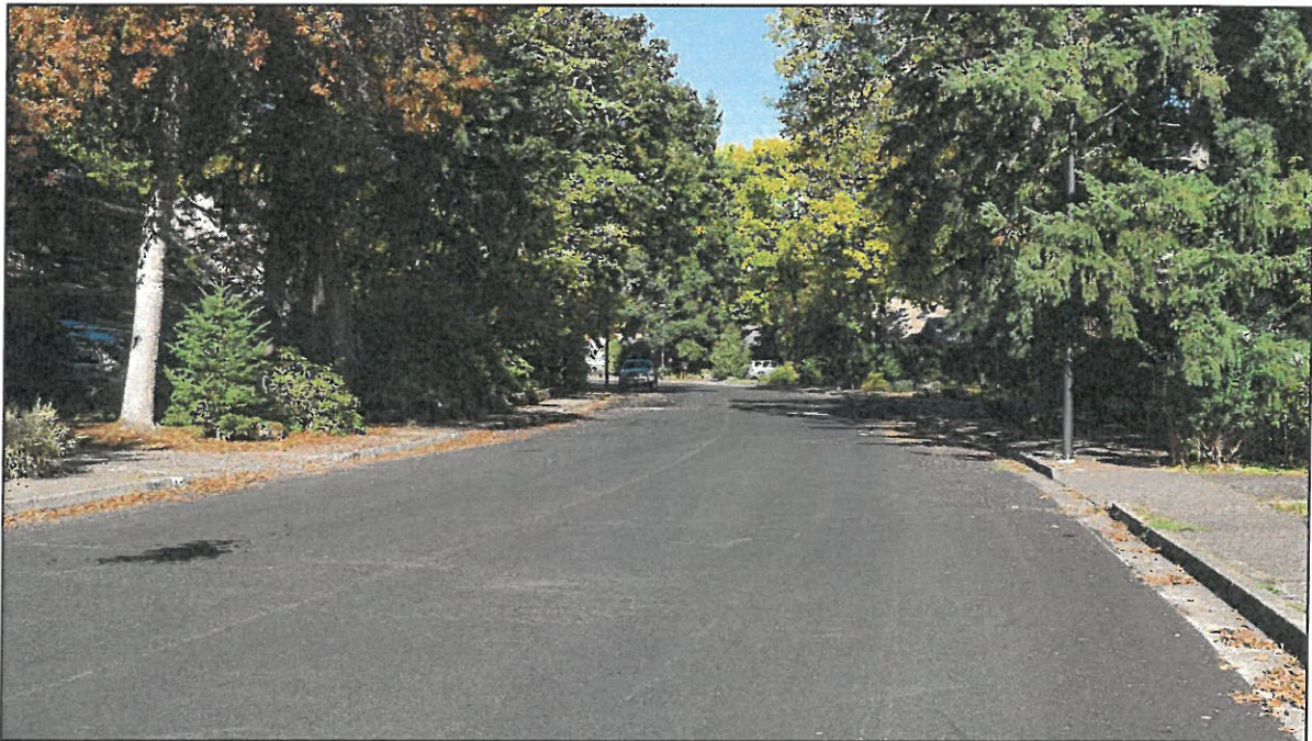
Completed Paving on Windsor Circle
