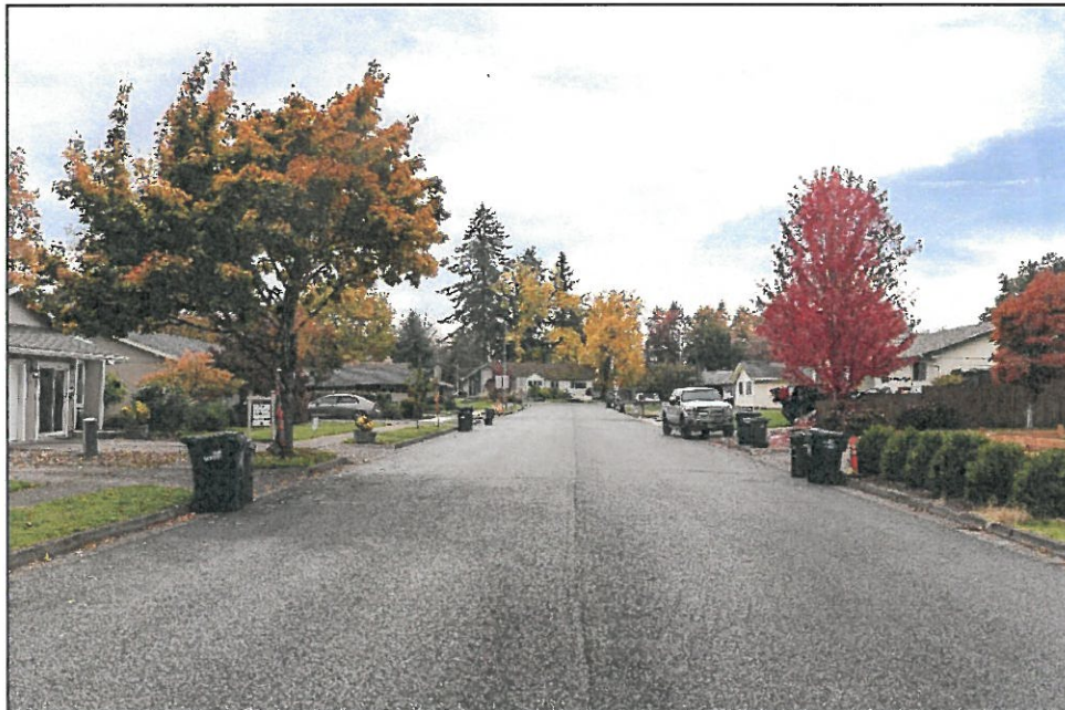
Completed Paving on Laurelhurst Drive
