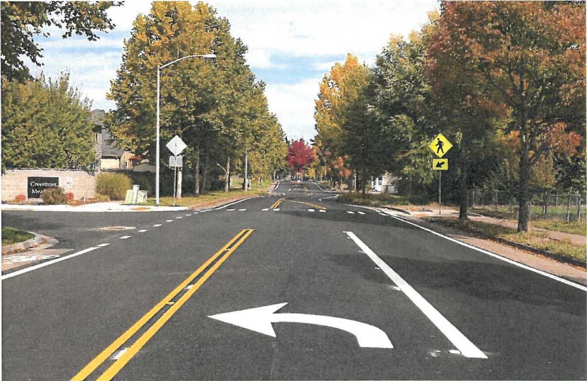
Completed Paving on Terry Street
