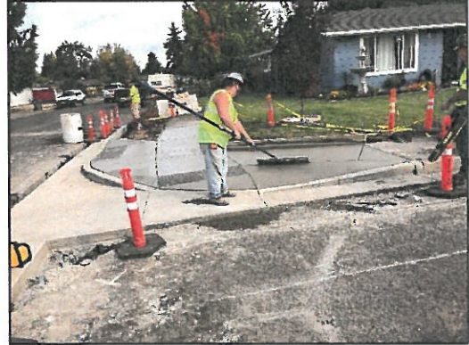
ADA Ramp Under Construction on Laurelhurst Drive
