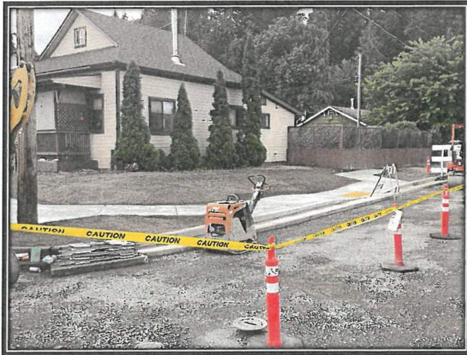
G Street & Chestnut Ave. Street, Curb, & Sidewalk Repair
