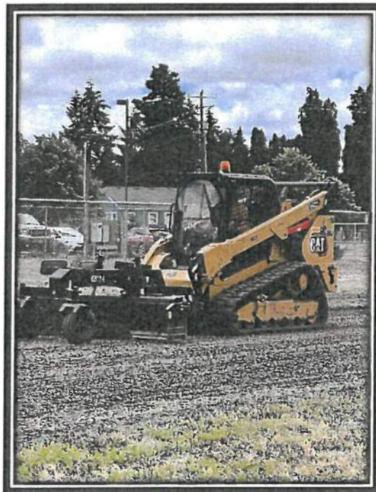
Grading gravel parking lot at N. 12 th Street
