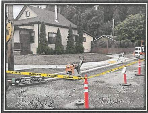
Street & sidewalk repair
