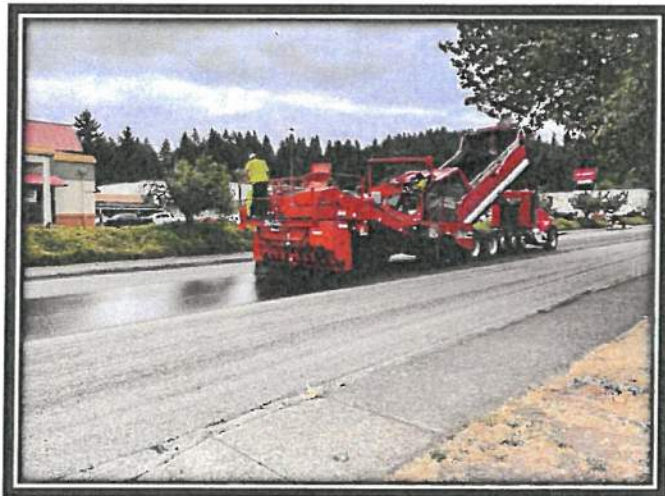
Chip Sealing Gateway Blvd.
