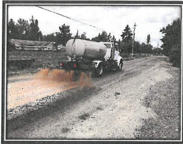
Dust abatement application on Lane Street
