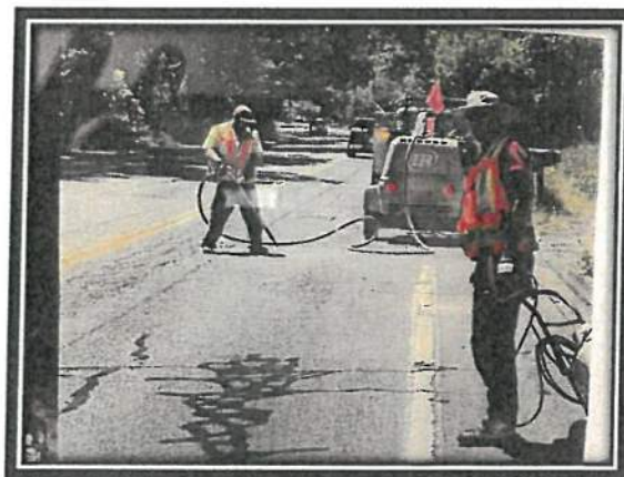
Crack sealing North River Road
