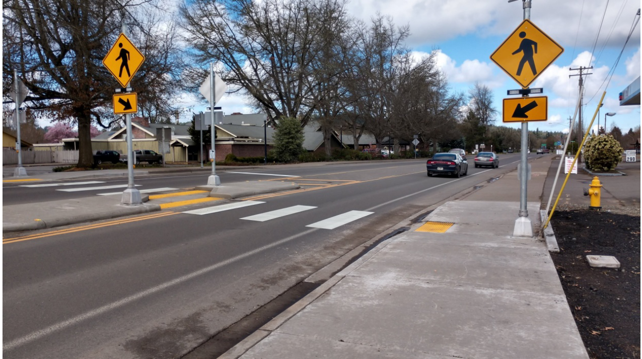
Row River Road – New Pedestrian Crossing
